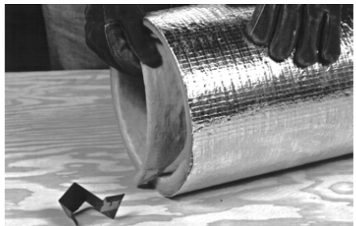
Fig. 7-2C. Using shiplap cutter to make female shiplap. Cutter is positioned to cut into inside of duct wall.
