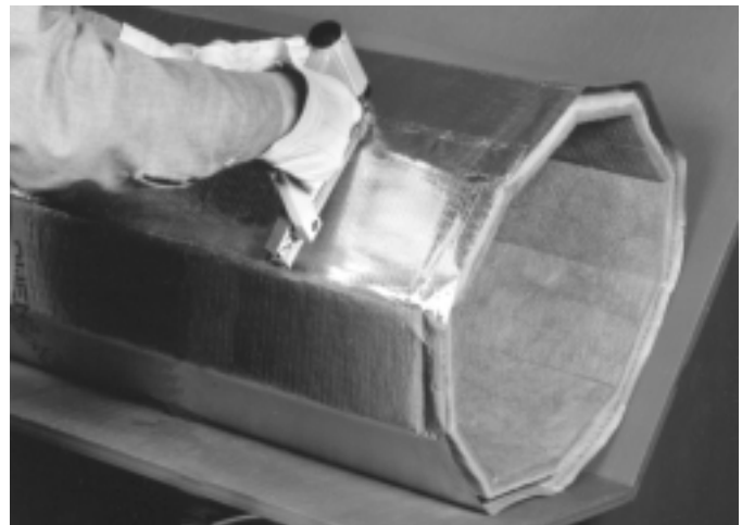
Fig. 3-34B. Stapling longitudinal joint of ten sided duct.
