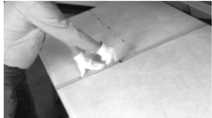
4. From there, measure 10" (254mm), same as second inside duct dimension, + add-on allowance of 1\frac{3}{8}" (35mm), total 11\frac{3}{8}" (289mm). Draw fourth corner groove centerline.
