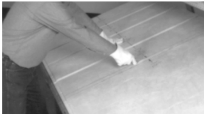
10. Using straight knife, cut along fourth corner break line through insulation only. Do not cut through or score the facing.
