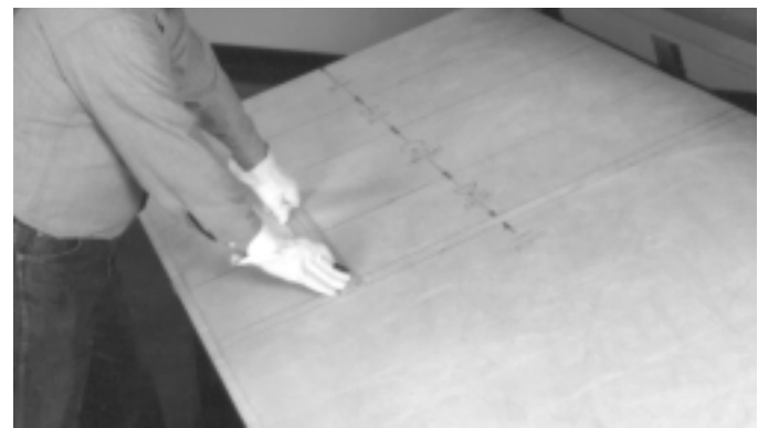
5. From there, measure 1\frac{3}{8}" (35mm) and draw line locating edge of closure flap. The board is now ready to be grooved. See next page.
