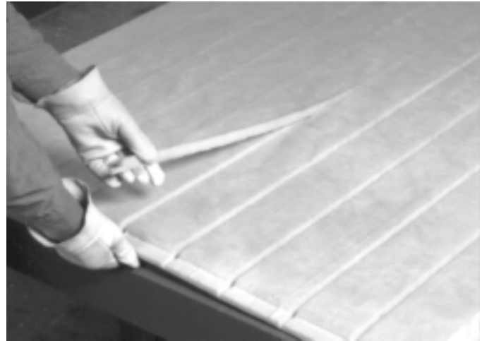
Fig.3-34A. Removing scrap from grooved duct board.
