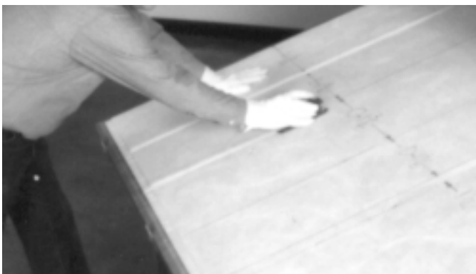
8. Rotate modified shiplap tool end for end (or use next sequentially numbered tool) and cut along second corner break centerline so right side of panel #2 is cut straight and shiplap is on left side of panel #3. Lift board slightly and remove groove scrap.
