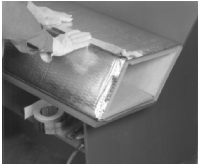
2. Fold to form the duct section, making sure ends are flush and seated properly in the shoulder of the shiplate edge.
