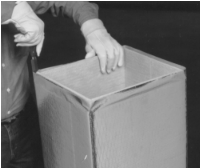
1. Slit facing flaps back at corners, making sure you do not cut below the male shiplap shoulder or into inside duct surfaces.
