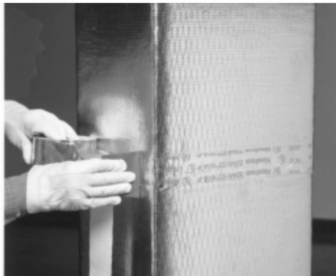
4. Complete closure of circumferential joint with UL 181A listed closure. (Pressure-sensitive tape shown above.) Duct board surface must be clean and dry.
