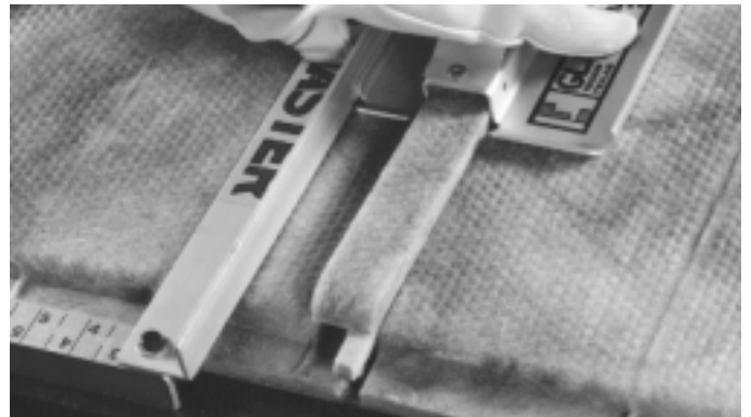
4. Place corner grooving tool (modified shiplap or V-groove) along guide edge of squaring tool and cut first corner groove. Remove groove scrap.
