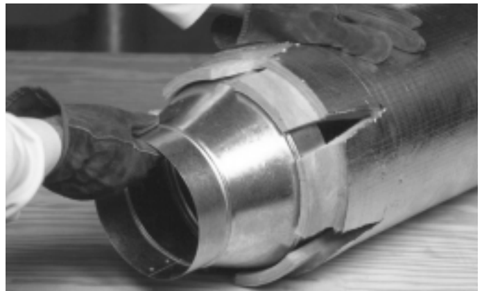
Fig. 7-5B. Inserting metal reducer into preformed round duct.
