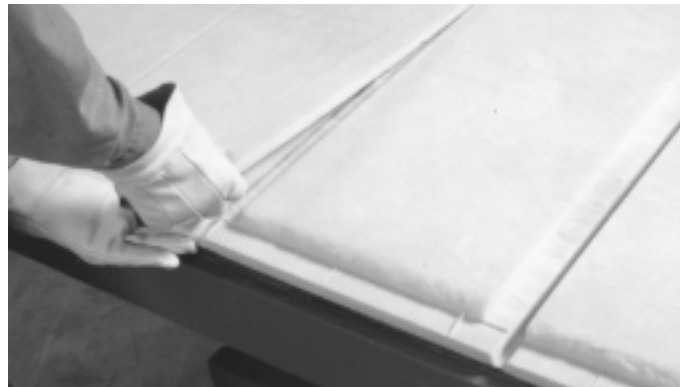
Fig. 2-11. Remove groove scrap. Confirm dimensions. The board is now ready for assembly and closure of a straight duct module, or for fabrication of a fitting.
