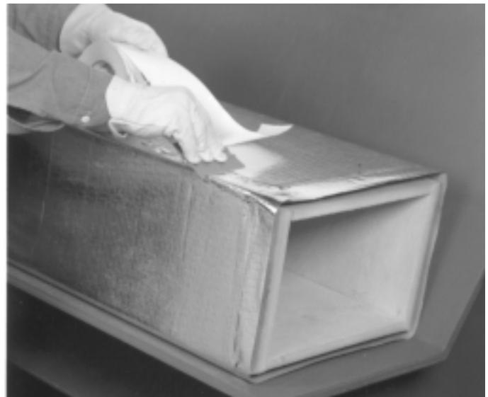
4. Complete the longitudinal seam according to procedures shown in Section IV, CLOSURE, page depending on the approved closure method chosen. (Pressure-sensitive tape shown above.)
