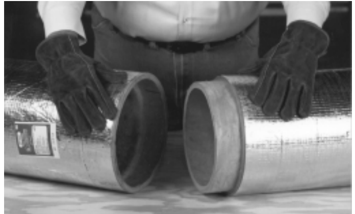
Fig. 7-2A. Preformed round duct sections are joined with male and female shiplaps. Joints are taped; staples are not required.
