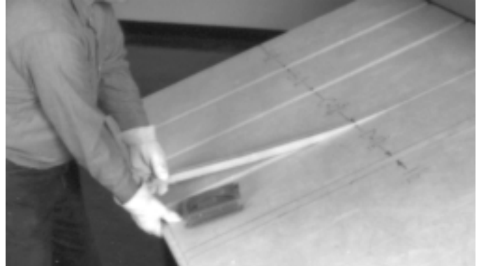
9. Rotate modified shiplap tool back to position in step 7. Cut along third corner break centerline so right hand side of panel #3 is shiplapped and left hand side of panel #4 is cut straight. Remove scrap.
