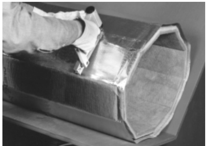
Fig. 2-32B. Stapling longitudinal joint of ten sided duct.
