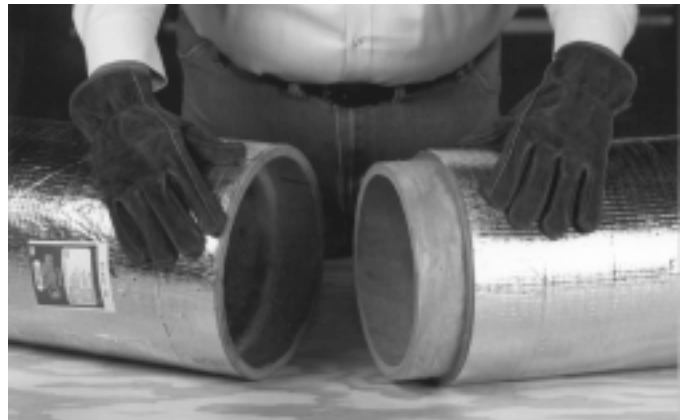
1. Performed round duct sections are joined with male and female shiplaps. Joints are taped; staples are not required.
