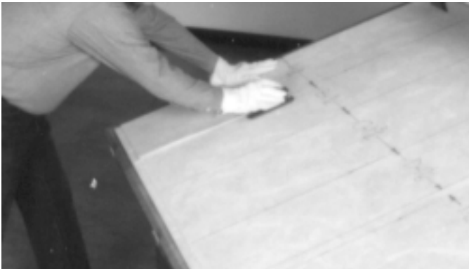
7. Cut along first corner centerline with modified shiplap tool so shiplap is on right side of panel #1 and left side of panel #2 is cut straight. Remove groove scrap; this is easily done if board is lifted slightly.
