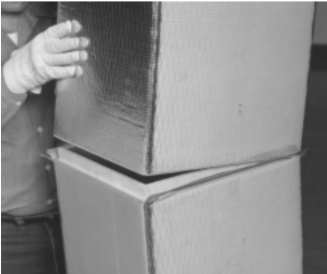
2. Push the two modules together. Make sure male and female shiplaps are tightly fitted together.
