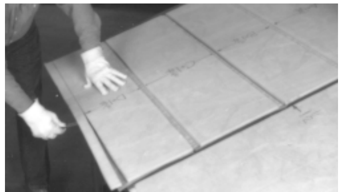
11. Using straight knife, cut through insulation and facing along last line - the line representing outer edge of closure flap. Peel insulation from flap. The board is now ready for assembly and closure to form a straight duct module or fitting.
